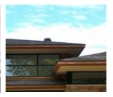
Gutters shall be built of metal of a color and finish that blends with the finish color scheme. Gutters shall be half-round or rectangular and downspouts shall be circular or rectangular.
