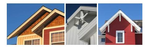
Fascia detail must have a minimum dimension of 8-inches nominal unless otherwise approved for design merit. The material used must fit the aesthetic of the structure. As an alternative, exposed rafter tails and entry accents are encouraged if appropriate for the architectural style.
