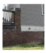
Foundation walls shall be exposed a maximum of 12-inches above the ground. Exposed foundation walls shall be built of brick, cast concrete, trimmed with horizontal members, or as otherwise approved by the DRC. Concrete foundations exposed more than 18-inches above grade must have an architectural finish (texture, pattern and/or color).
